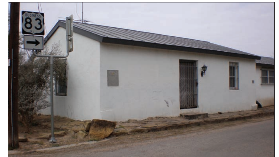
Figure 2.27: Historic customs house. Trevino Street.
